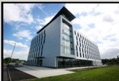
EXAMPLE OF A HOTEL IN MANCHESTER BUILT IN ITS ENTIRETY WITH SHIPPING CONTAINERS.
